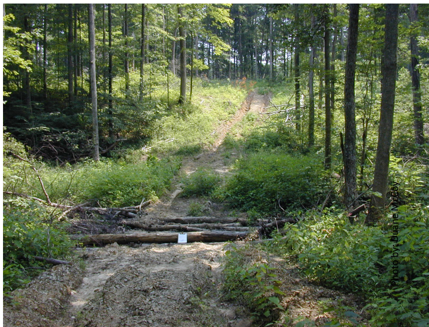
There are multiple issues on this skid trail and stream crossing. Logs used as corduroy to cross stream were not removed after the harvest was closed out, and there are no diversions on the skid trail coming down the hill. Lack of diversions and rutting are ensuring that all runoff is being funneled right into the stream.
