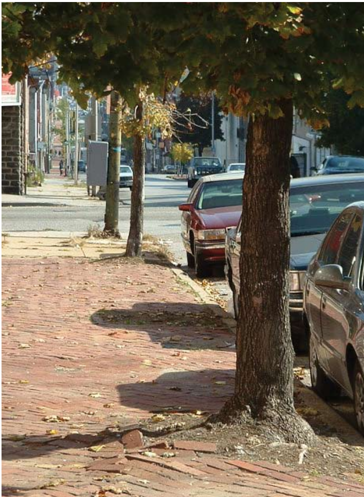
Figure 9. A common infrastructure conflict results in tree roots lifting or cracking pavement due to inadequate setbacks between trees and pavement.
