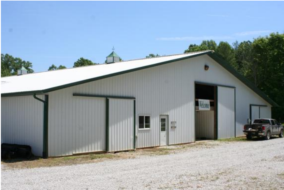
Horse barn with arena and stalls
