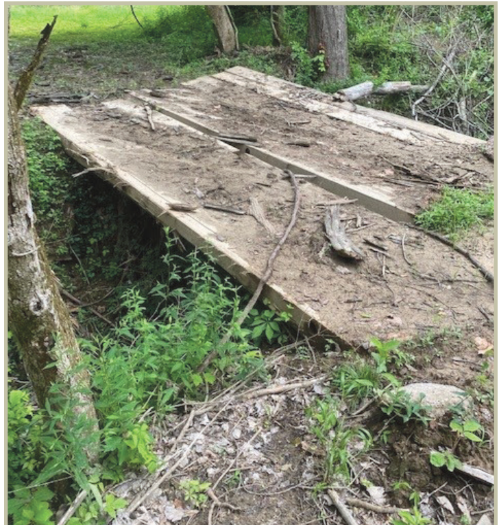
A temporary bridge can greatly reduce impact to streams during a timber harvest.
