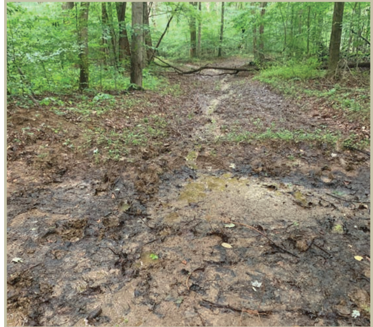
A poorly designed and implemented waterbar breached at the top of a hill allows runoff to continue down the hill on a skid trail, picking up volume and velocity, which increases erosion. Photo by Jennifer Sobecki
