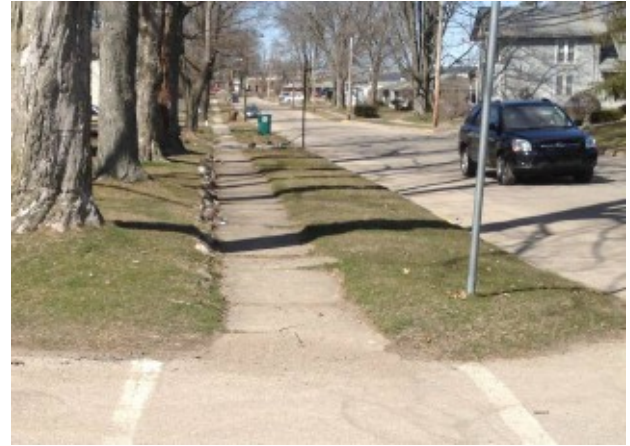
Example of lack of DW at blended transition
