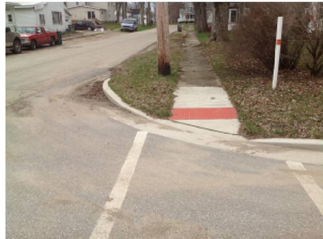
Example of proper application of detectable warning at blended transition
