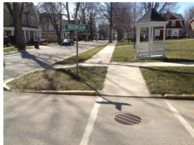
Example of lack of DW at curb ramp. Also example of undesirable grate within the PAR of the adjacent crosswalk (See 6.9)
