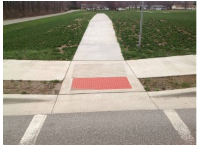
Example of parallel ramp with compliant lower landing/change of direction to enter crosswalk, however DW is not full width.
