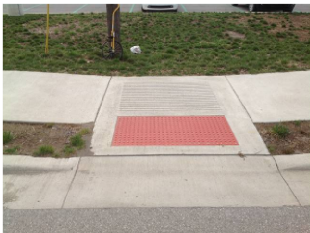
Example of DW that does not extend full width of curb ramp
