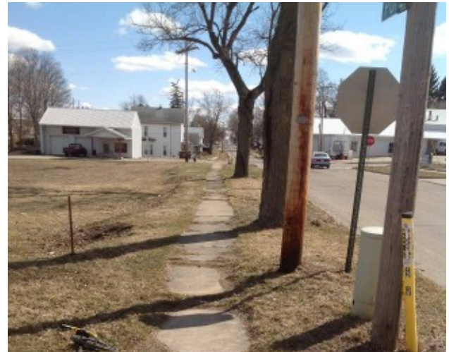
Example of sidewalk width narrowed by overgrowth
