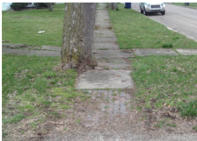
Example of obstruction of required 48" minimum clear width by tree
