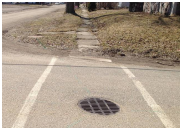
Example of evidence of ponding at ramp and non-compliant grate within crosswalk PAR
