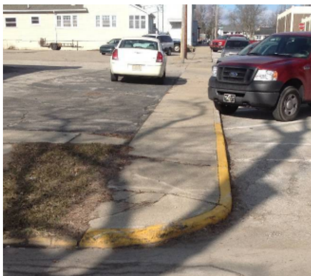
Example of obstruction of required 48" minimum clear width by vehicle overhang of adjacent parking
