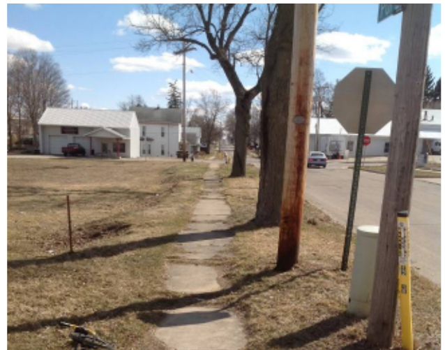
Example of sidewalk width narrowed by overgrowth
