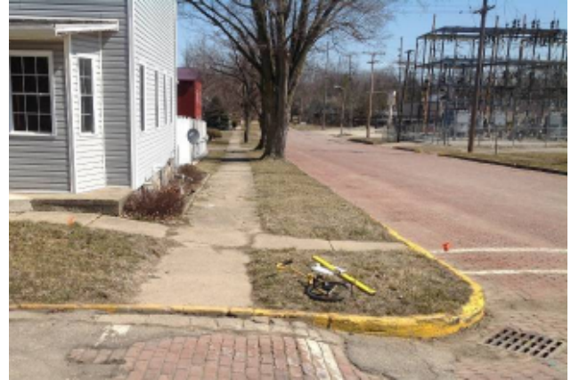
Example of non-compliant lip at bottom of curb ramp
