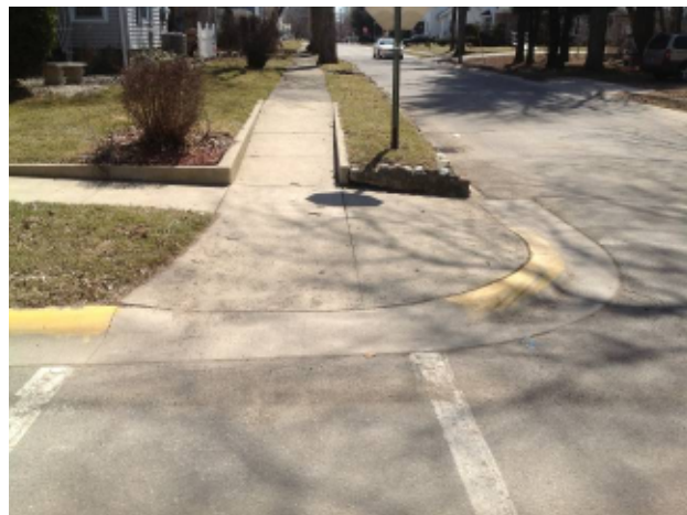
Example of compliant flare and top landing between two perpendicular ramps, but is lacking detectable warning.
