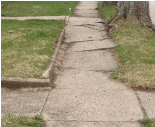
Example of displacements and cracking of sidewalk at existing tree
