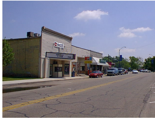
The midtown area has developed an entertainment-like theme. It is suggested that this theme be embraced and promoted to develop a year-round regional draw.
