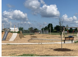
Cavalier Park Progress
