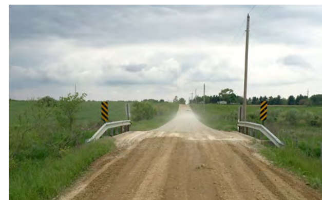
Bridge over a ditch on 20 A Road that will need to be widened to include a trail
