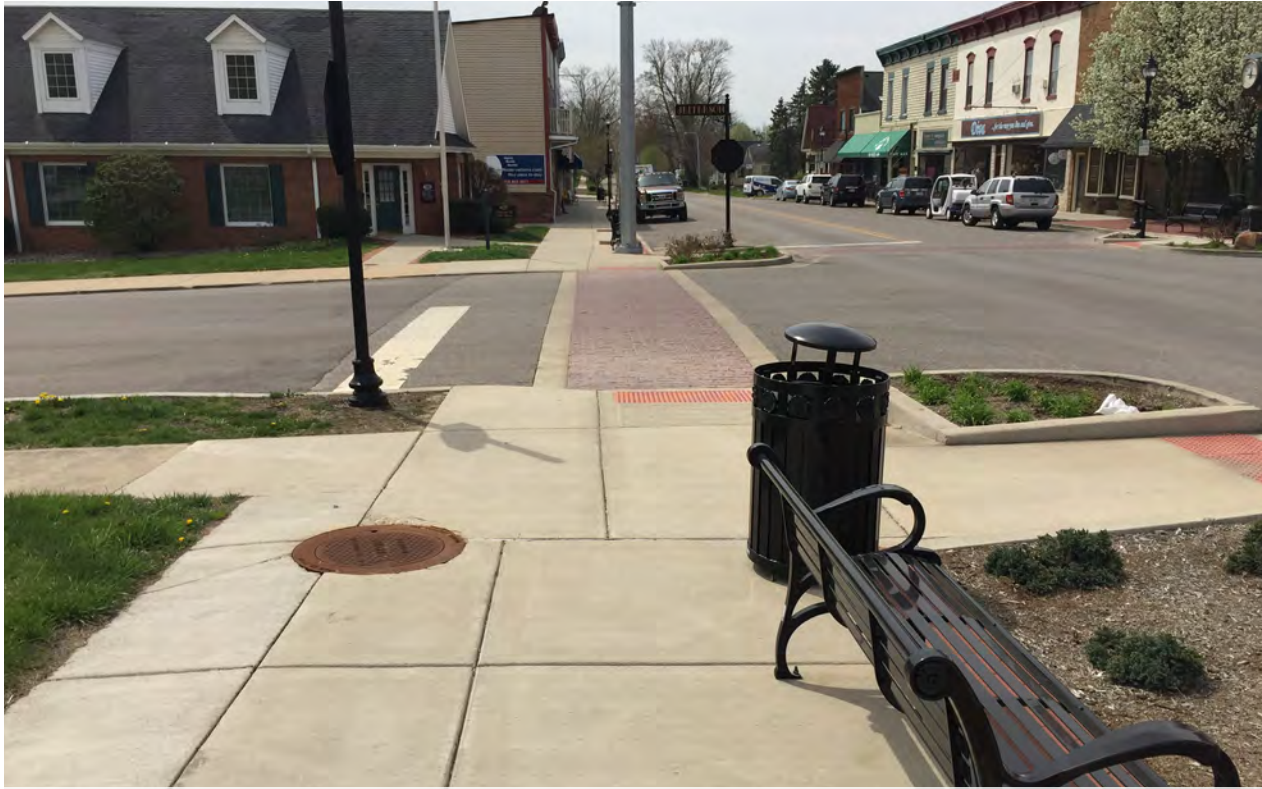
Downtown Culver, featuring ADA crosswalks, wider sidewalks, and standard benches and trash receptacles.
