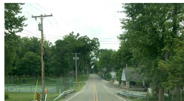
Narrow right of way and utilities along East Shore Dr will make a roadside trail difficult
