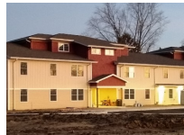
Finishing Touches at Sand Hill Farm
