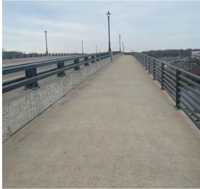
US-12 bridge over Trail Creek – Michigan City, IN
