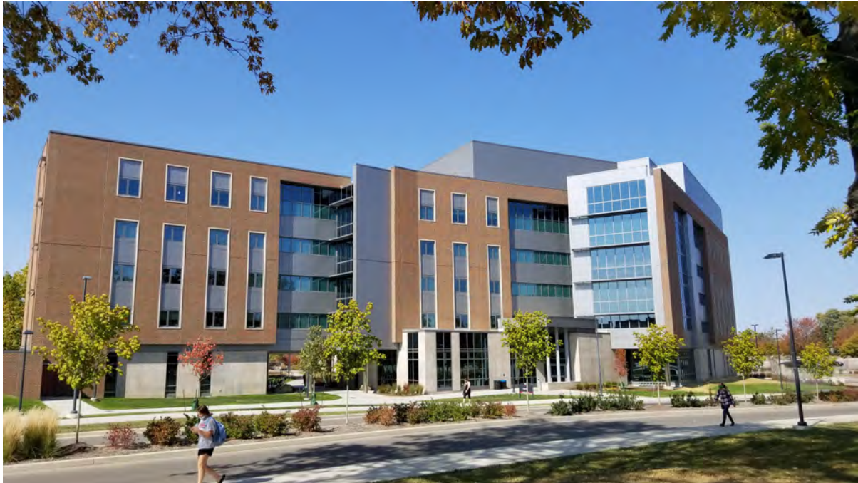
North Residence Hall
