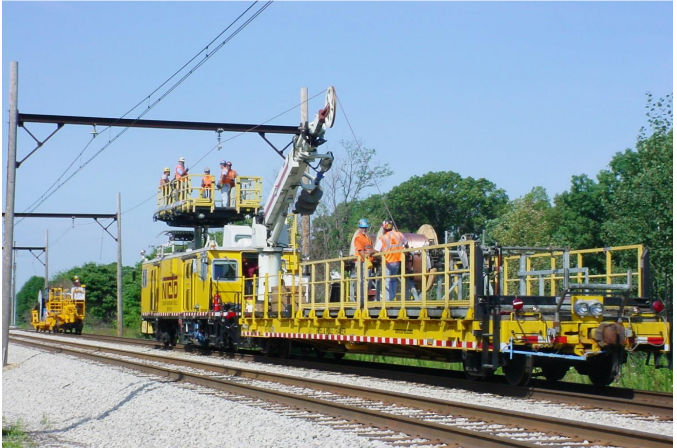
Line and Signal crews install new catenary wire.
