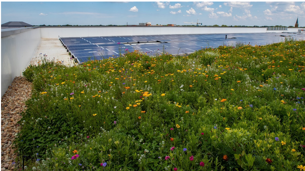
Health Professions Building Green Rooftop
