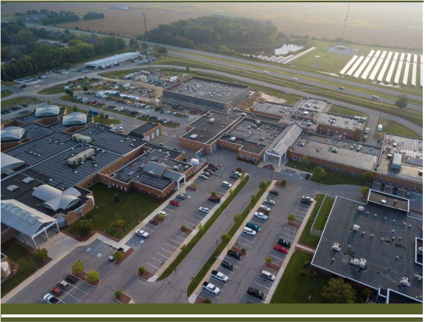
Solar Panels at Corrections Facility
