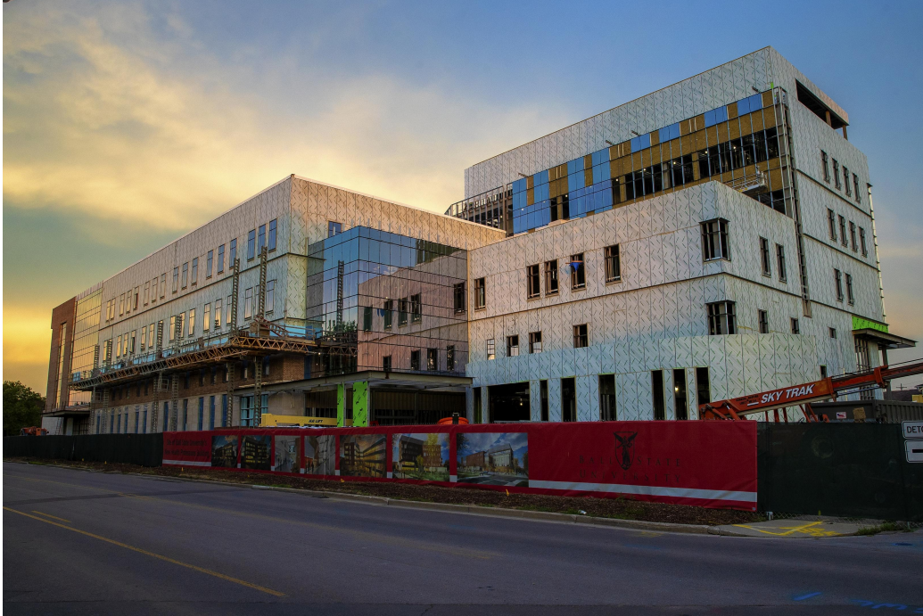
Health Professions Building construction
