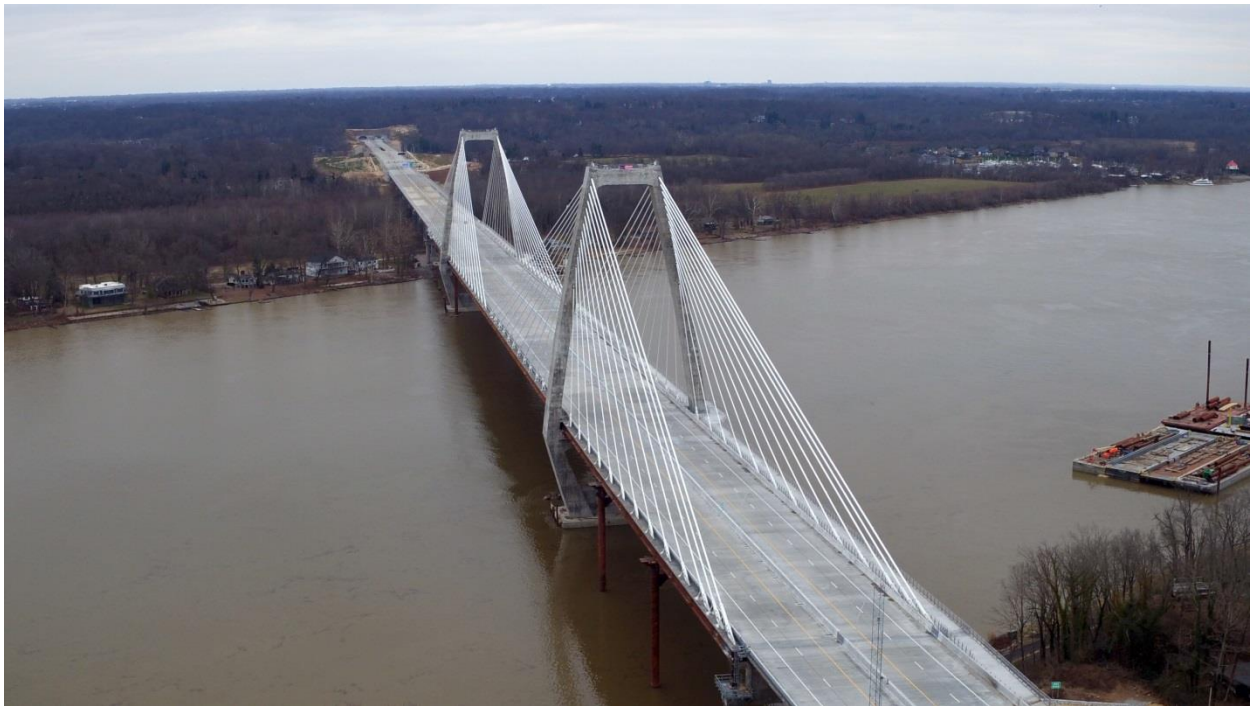
The Lewis and Clark Bridge spans the Ohio River and connects Indiana State Road 265 with Kentucky State Highway 841. (Photo courtesy of INDOT)
