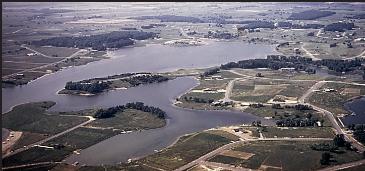
Construction of Lakes of the Four Seasons
