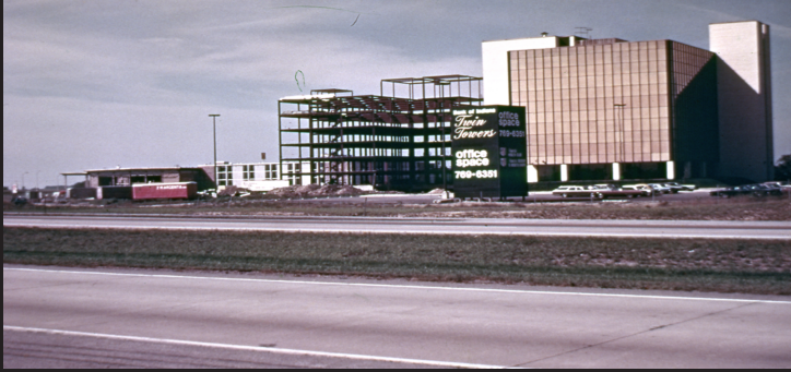
Construction of Twin Towers
