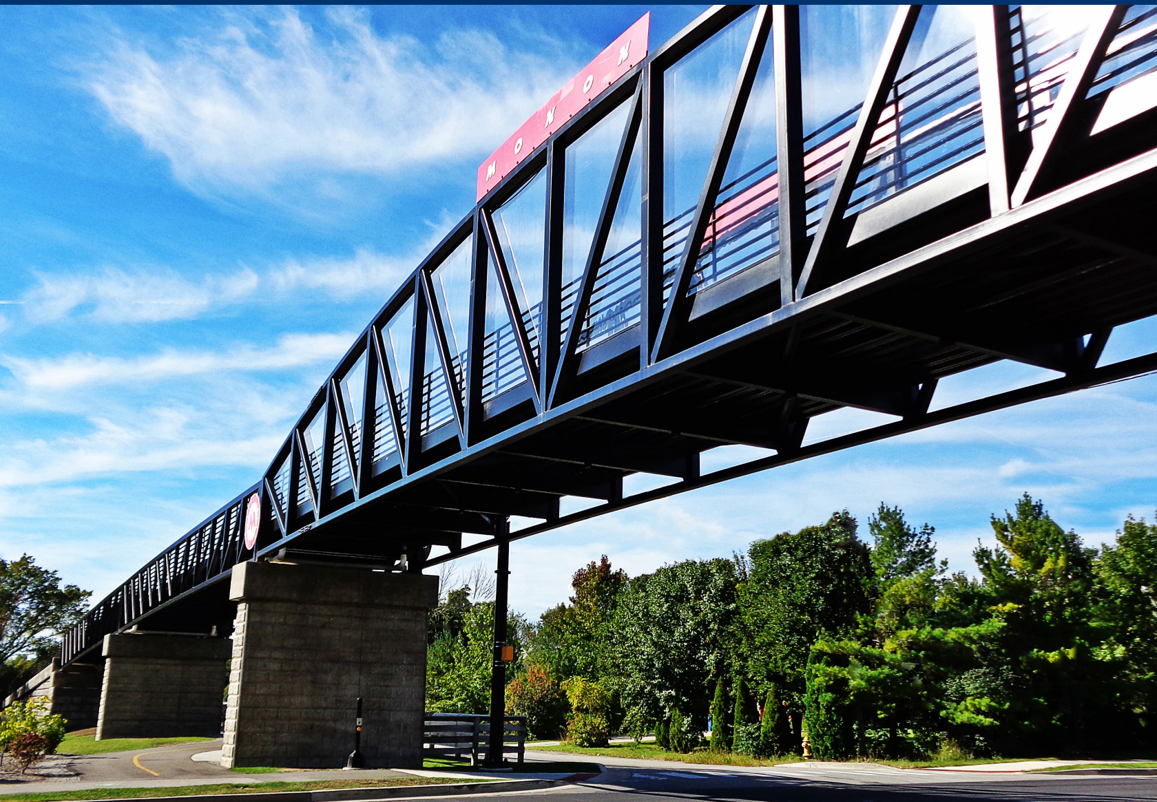
Monon Trail Pedestrian Bridge Photo courtesy of Dustin Teachnor
