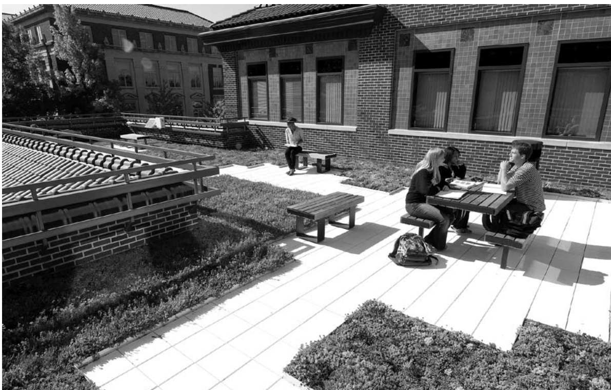
Schleman Hall "green roof"
