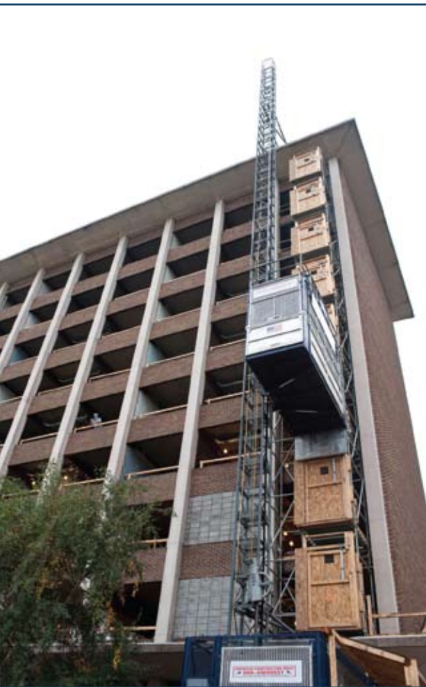
Sandison Hall renovations
