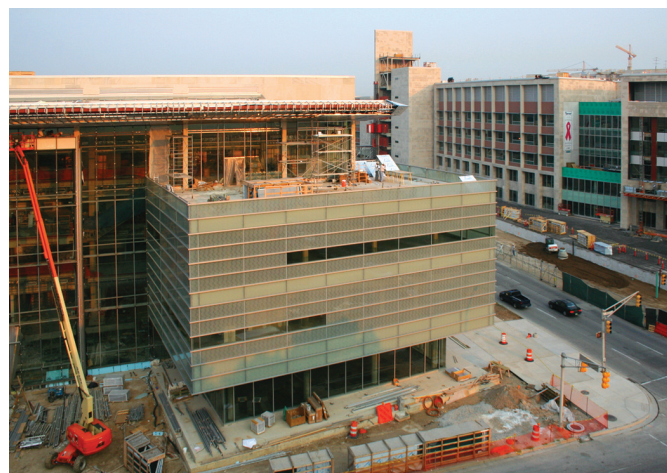
Campus Center construction, IUPUI
