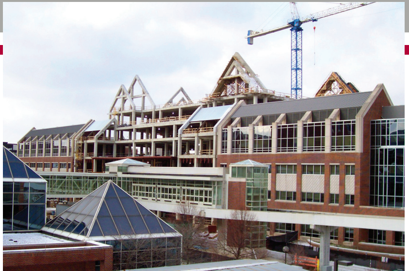
Research III construction, IUPUI
