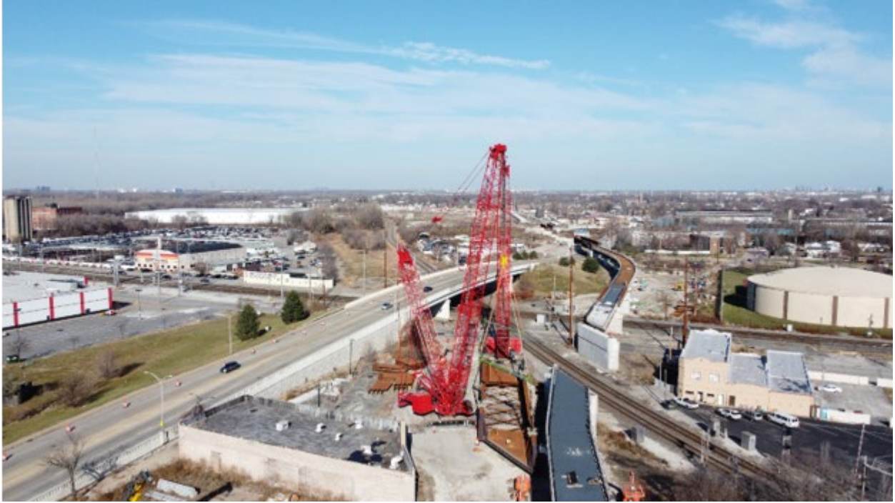
Metropolitan Steel assembling Bridge 110 in advance of setting the structure over the Norfolk Southern Railroad in Hammond, Indiana as part of the West Lake Project.
