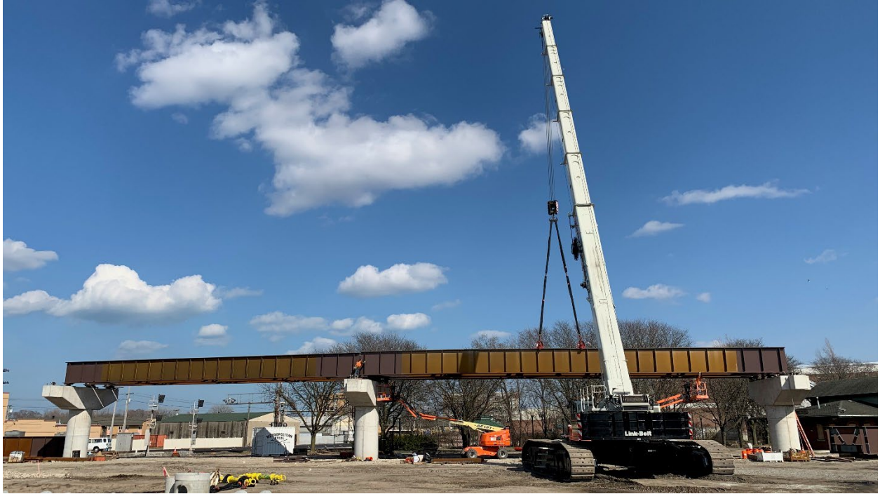
Metropolitan Steel setting a steel superstructure beam on the elevated structure for the new Monon Corridor through downtown Hammond, Indiana as part of the West Lake Project.
