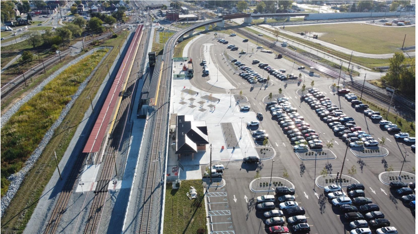
Aerial view of the new Hammond, IN Gateway Station on opening day, October 18, 2024. Construction of this new station marked a milestone in the West Lake Corridor project.
