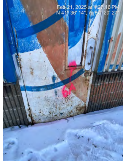
Sample #6 Exterior Caulk - Gray, flexible. On exterior and interior metal doors and windows
