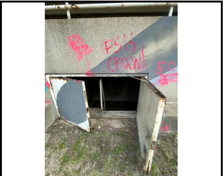
FS-16 (C) Crawlspace
