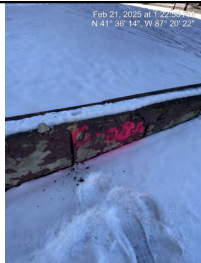
Sample #8 Concrete - Retaining walls
