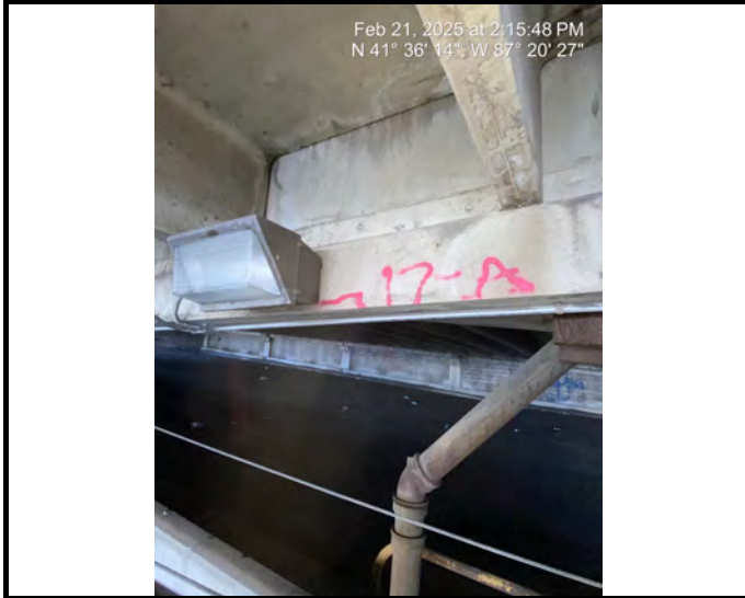
Sample #17 Heat Shield - Light Fixtures, along interior center wall
