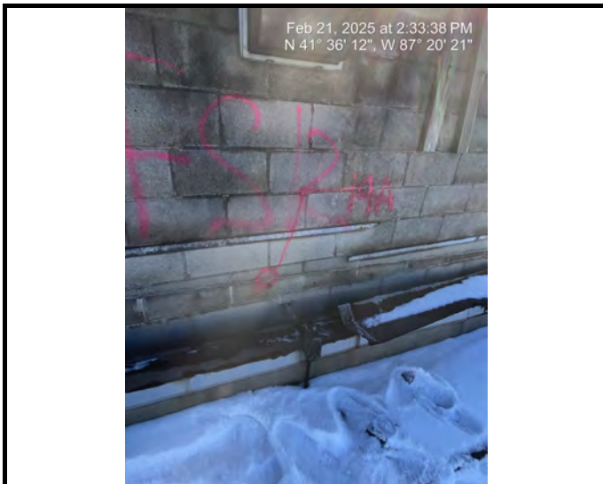
Sample #19 Exterior Caulk - On metal at roof parapets
