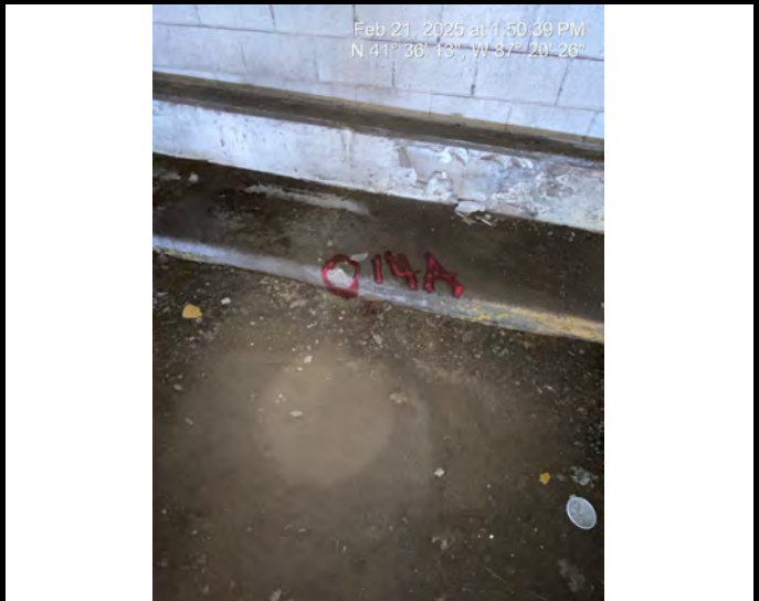
Sample #14 Concrete - Parking garage interior curbs
