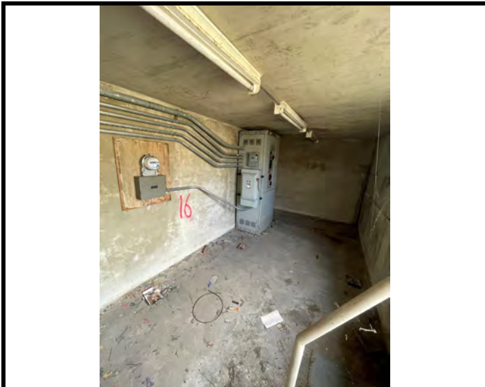
FS-16 (B) Crawlspace
