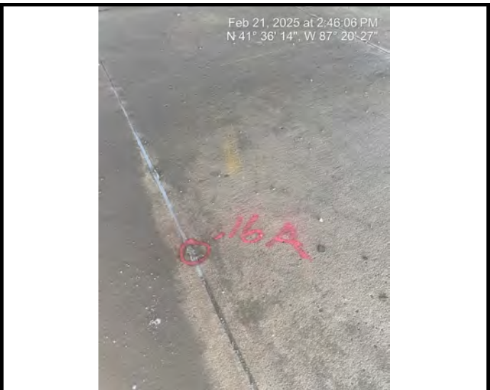
Sample #16 Interior Caulk - Gray, used as expansion joint in concrete paving
