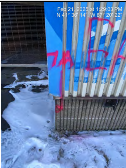
Sample #7 Brick Mortar - Exterior ridged gray brick w/mortar
