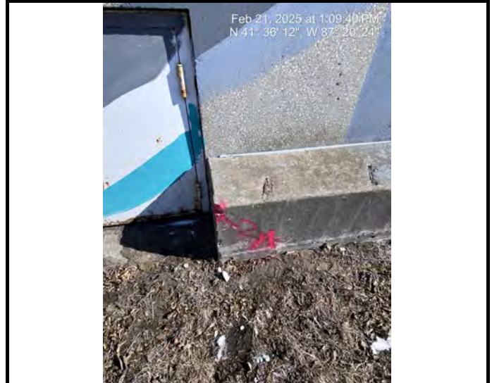
Sample #2 Concrete - Exterior footing, at base of building
