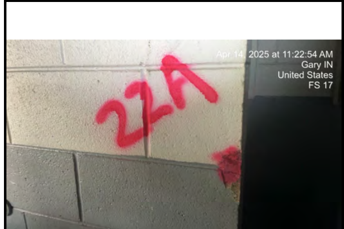
Sample #22 Block Mortar - Interior Wall Block with Mortar
