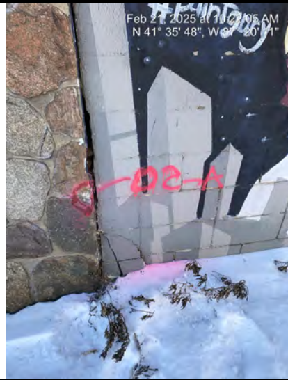
Sample # 2 Brick Mortar - Exterior Decorative Stone Façade
