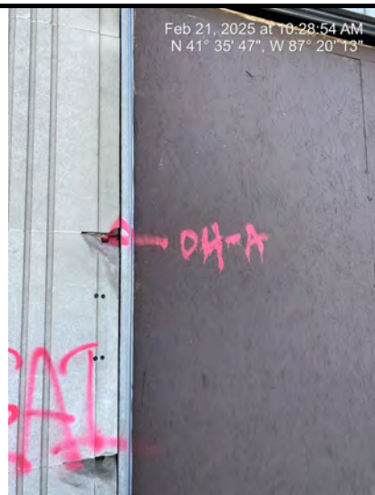
Sample # 4 Concrete - Exterior columns & beams w/mortar
