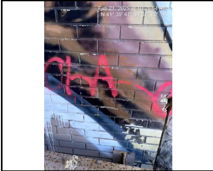
Sample # 1 Brick Mortar - Exterior glazed brick with mortar
