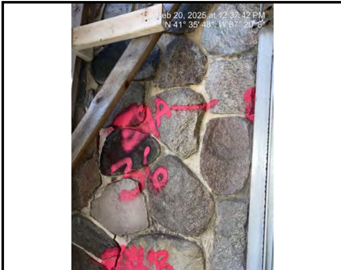
Sample # 36 Interior Caulk - Black/Gray, on metal door frame at east vestibule
