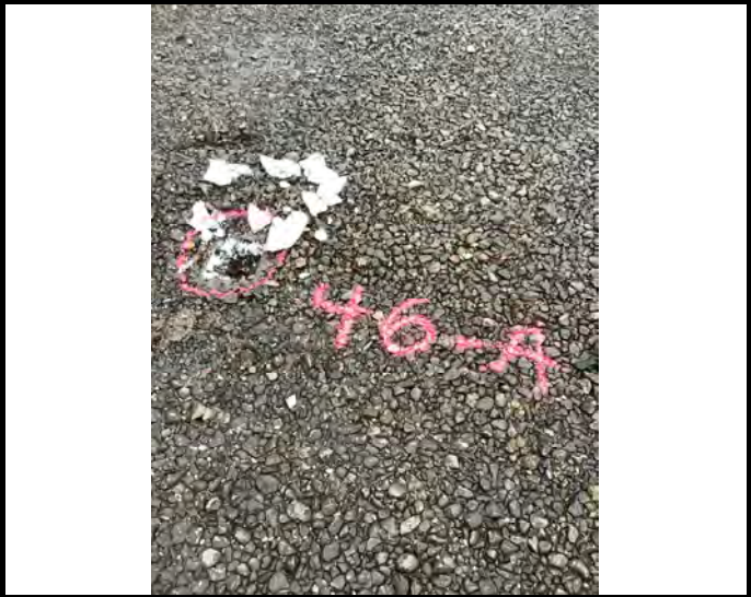
Sample # 46 Roofing Material - Flat Roof Material
