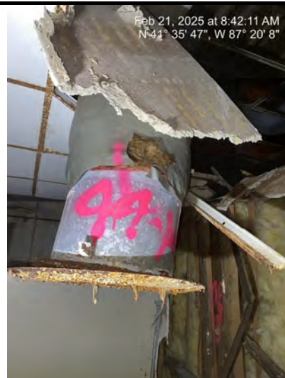
Sample # 44 Insulator - Fiberglass sound proofing
