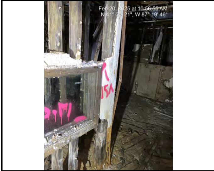
Sample # 15 Plaster - Skim & Base Coat Walls on Wall Board
