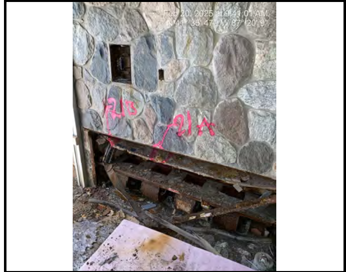
Sample # 21 Rolled In Insulation - Yellow fiberglass with thick tar Paper backing
