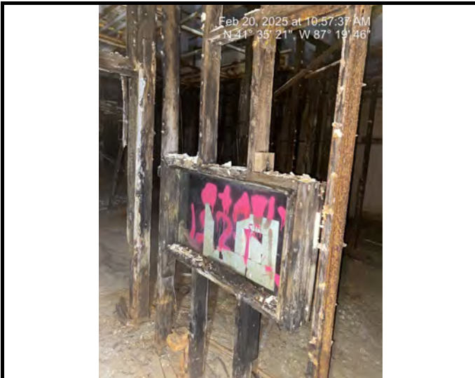
Sample # 17 Window Glaze - Gray, On wood frame of bathroom windows
