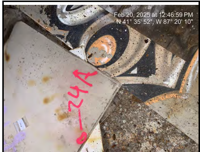
Sample # 24 Interior Caulk - Gray, on metal panels on floor
