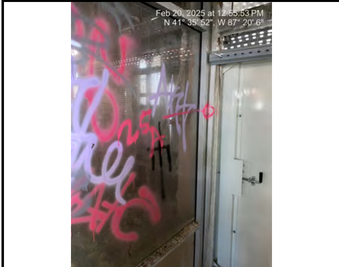
Sample # 25 Interior Caulk - Gray, flexible, on Metal door trim at west vestibule
