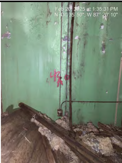
Sample # 42 Expansion Joint - Black , at joints between concrete slabs, behind caulk.
