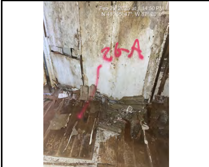
Sample # 26 Construction Adhesive - Yellow, behind wood paneling
