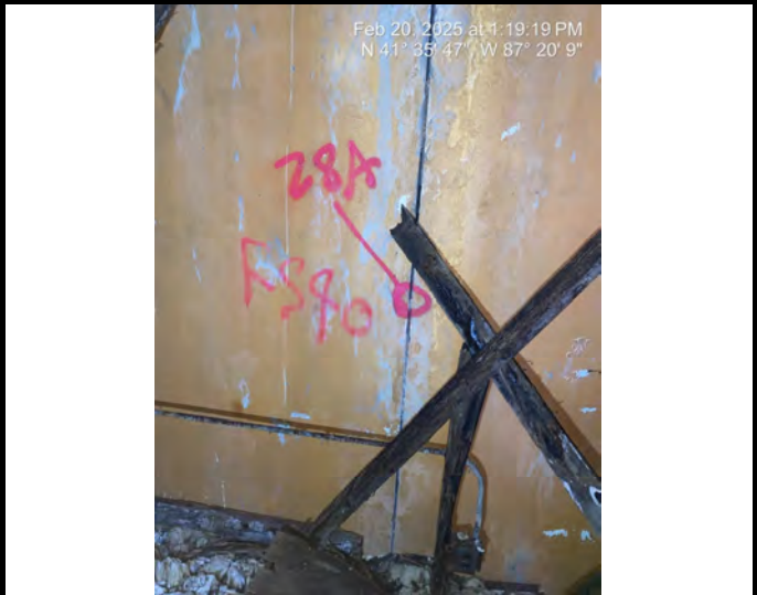
Sample # 28 Interior Caulk - Gray, between concrete slabs along north & east walls
