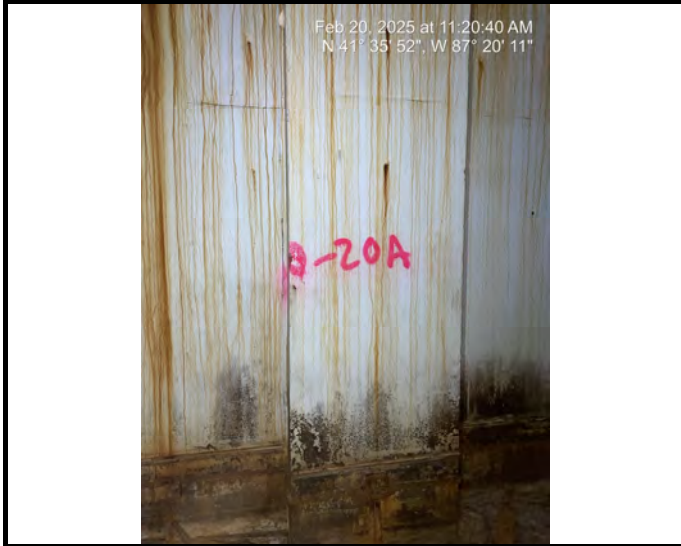
Sample # 20 Concrete - Foundation Walls
