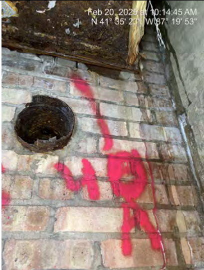
Sample # 40 Stack Cement - Chimney at Mechanical Exhausts
