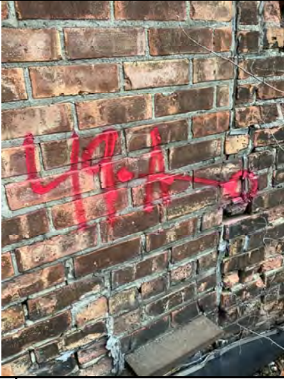
Sample # 49 Exterior Caulk- Brown - Used as a patch for brick mortar
