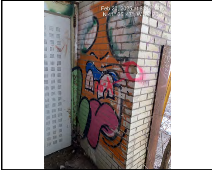
Sample # 6 Brick Mortar - Exterior, gray with white glazed brick
