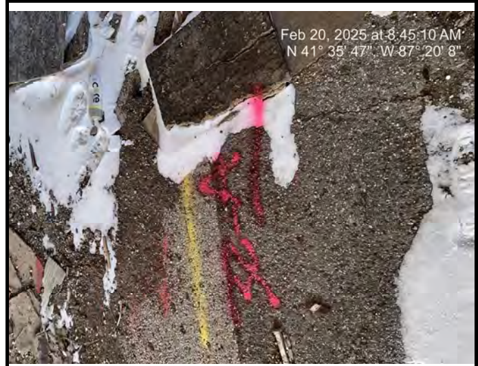
Sample # 32 Exterior Siding - Fiberboard, black, for sound proofing behind plaster
