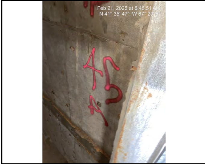
Sample # 45 Duct Insulation - Fiberglass/horse hair w/plastic
