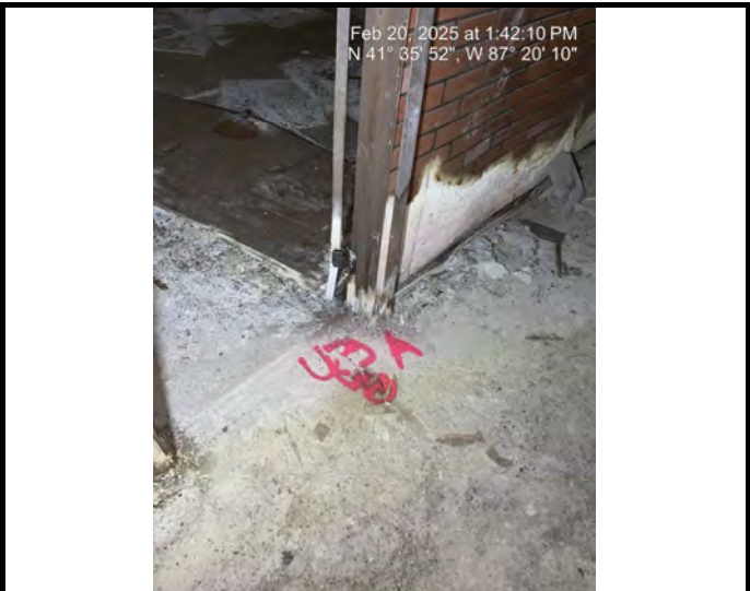
Sample # 43 Flooring - 12X12 Floor Tile with Mastic & Glue
