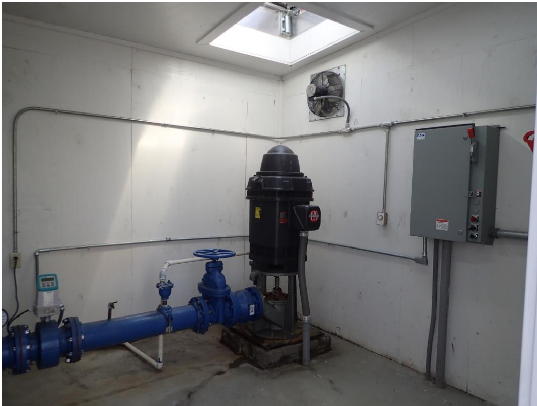
Interior view, Well #3, note overhead hatch for removal of pump
