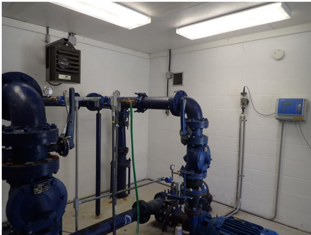
Interior view, booster station, note free chlorine measuring device on wall on right, one of two pumps in lower right
