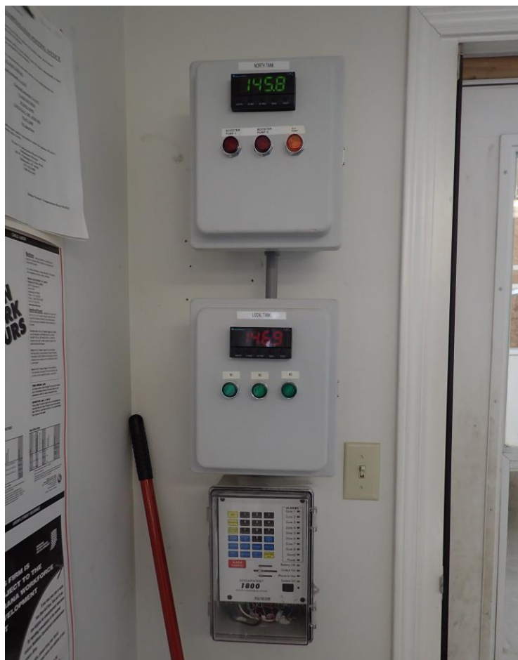
Tank levels, well, booster pump and chlorine feed Indicators, and alarm box at office
