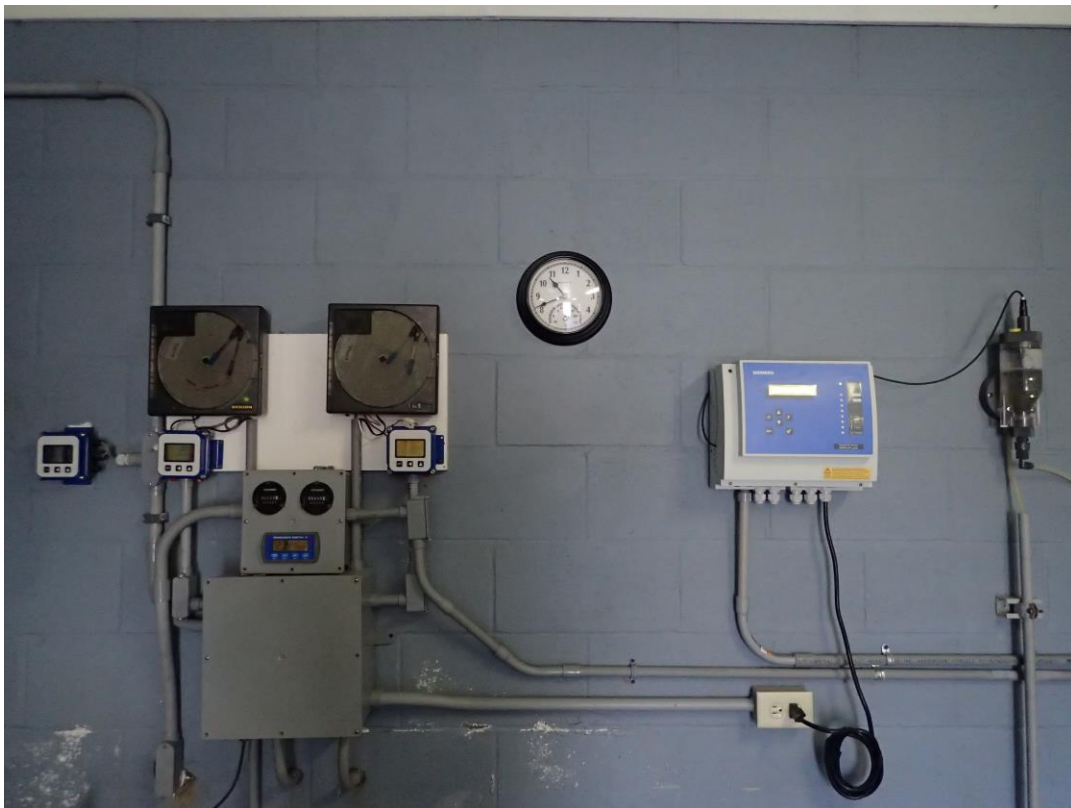
Interior chlorination building showing well (l) and chlorine residual (r) meters
