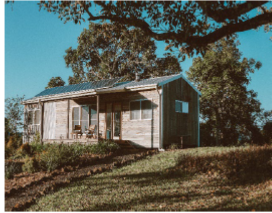
Figure 2. House with Solar Panels at Blue Knob Australia
