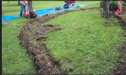
Build the berm with sod
