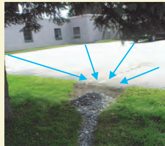
Estimating the stormwater that runs off streets, sidewalks, and parking lots can be tricky. It is best to visit the impervious area during a rain event to clearly see the extent of the drainage area.
