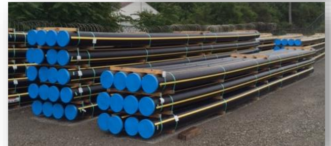
Bare Steel Replacement Project (Gary, Ind.)
