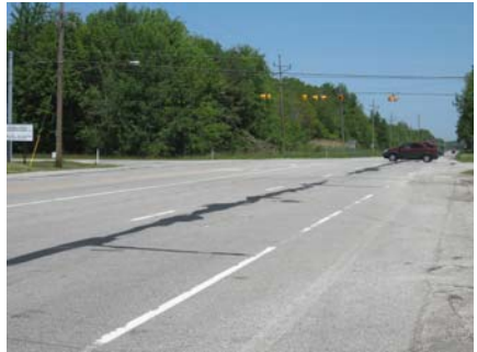
HMA Overlay: SR 212 From US 20 to US 12, Michigan City, Long Beach
