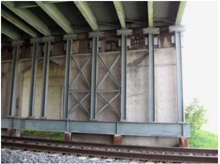
Bridge Repair; Temporary Support: SR 912 over Gary Avenue, Gary
