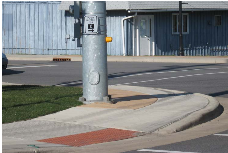
Major Pavement Project: Main Street from north town limits to south town limits, Hebron
