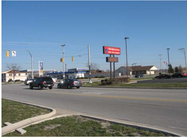
Intersection Improvement: 109 th Avenue at Randolph Street, Winfield
