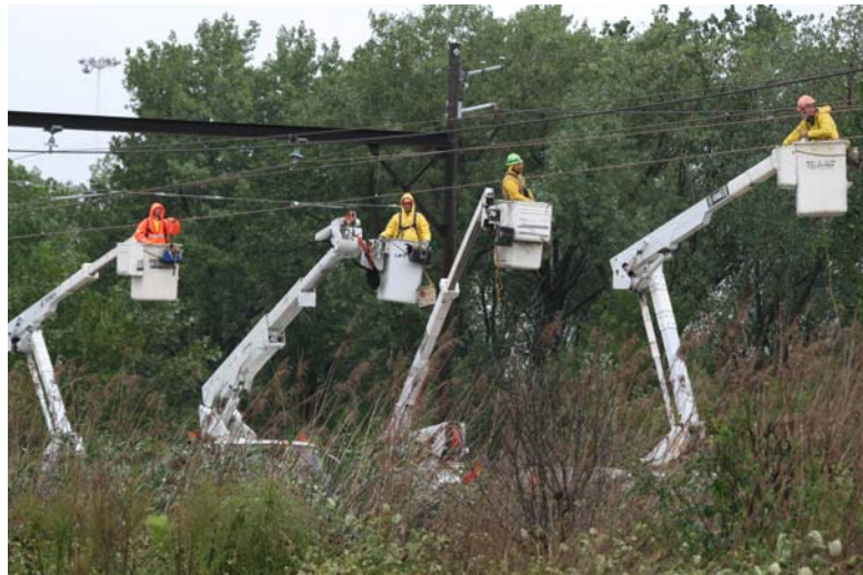
Replacement Catenary and Signal System, Northern Indiana Commuter Transportation District, (photos courtesy of Meade Electric)
