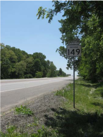
HMA Overlay: SR 149 from US 20 to Little Calumet River Bridge, Burns Harbor
