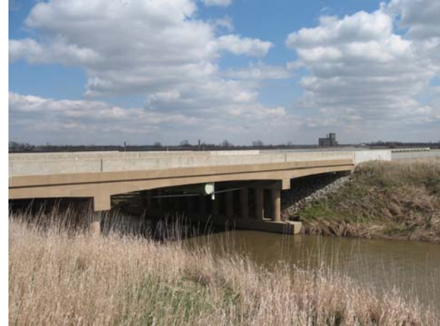
Bridge Repair: US-41 over Singleton Ditch, Lake County
