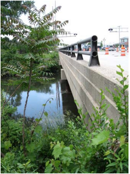
Bridge Repair; Temporary Support: SR 312 over Indiana Harbor Canal, East Chicago
