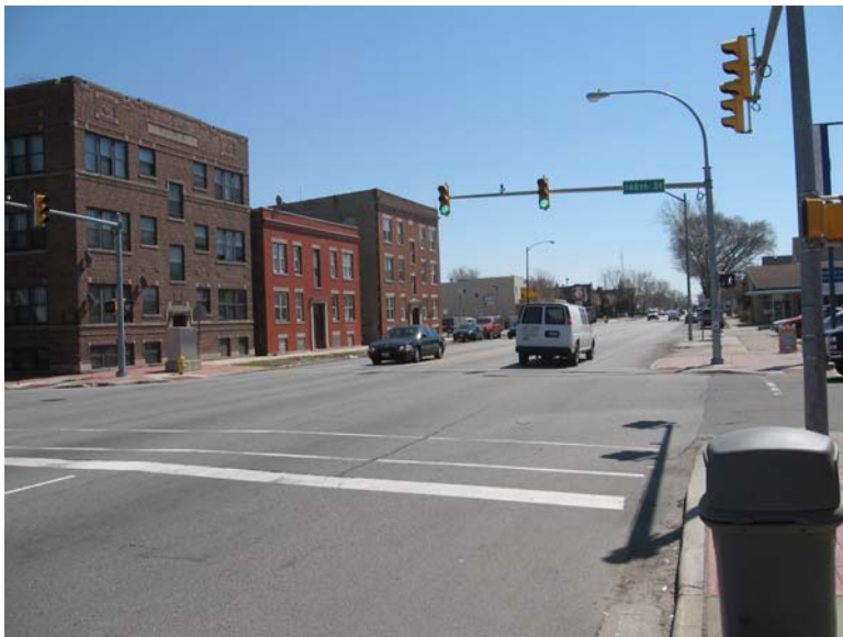
Road Resurfacing: US-20 from US-12 to SR-152, East Chicago
