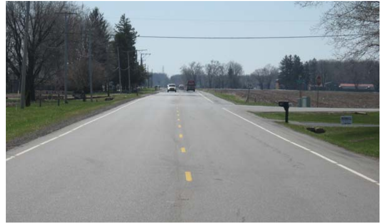
Resurfacing: SR-39 from US-6 to SR-2, LaPorte
