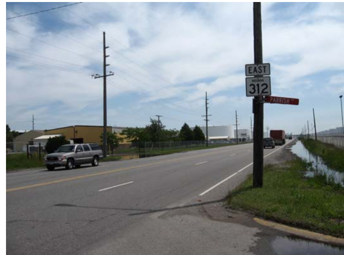
Asphalt Resurface: SR312 from Parrish Ave. to Cline Ave., East Chicago
