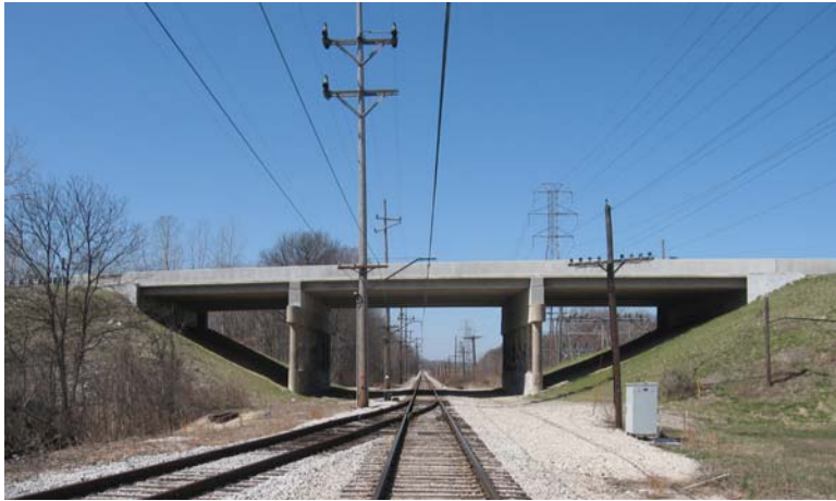
Bridge Superstructure Replacement: SR-212 over NICTD tracks, Michigan City
