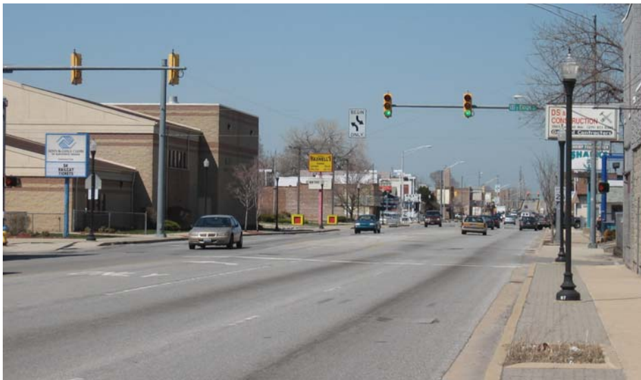
Pavement Replacement & Signal Modification: US-41, Hammond
