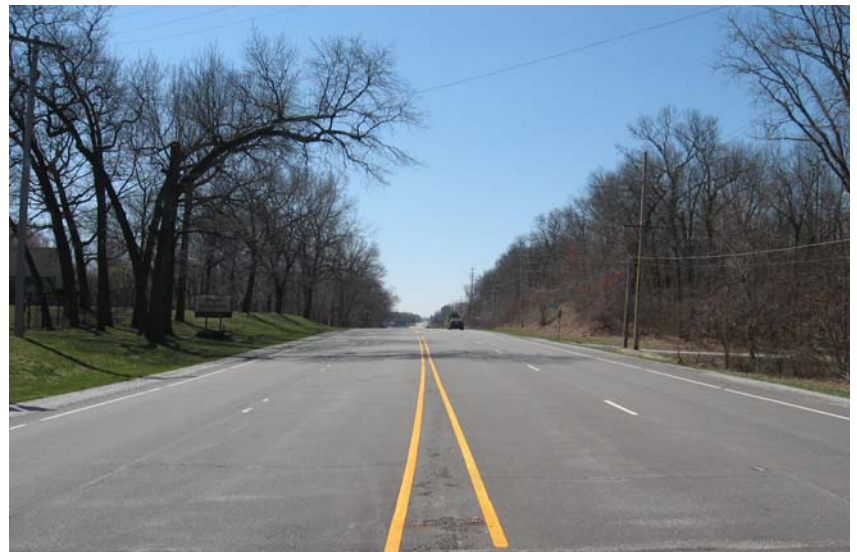
Road Resurfacing: SR-212, Michigan City
