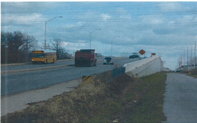
U.S. Highway 6 & 37 th Avenue bridge over railroad Hobart/Lake Station
