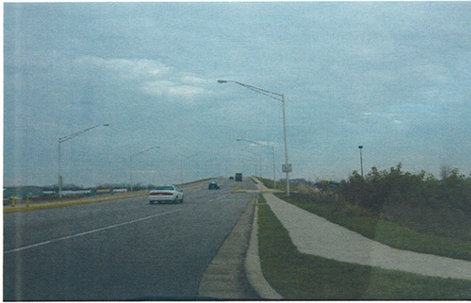
Calumet Avenue overpass north of U.S. Highway 30 Dyer
