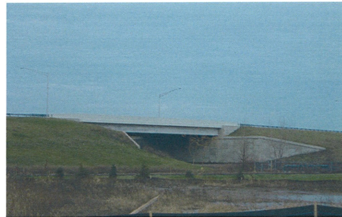
Calumet Avenue over railroad looking northwest Dyer
