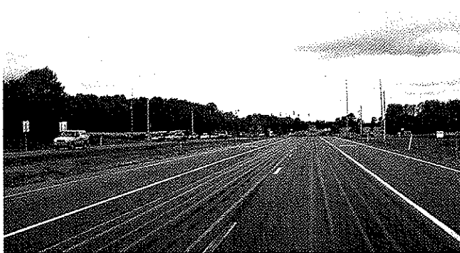
S.R. 49 Resurfacing – Porter County
