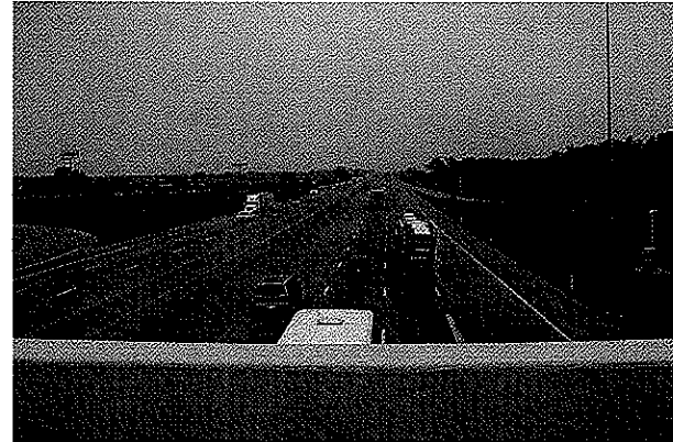
I-65 Lane Widening – Lake County
