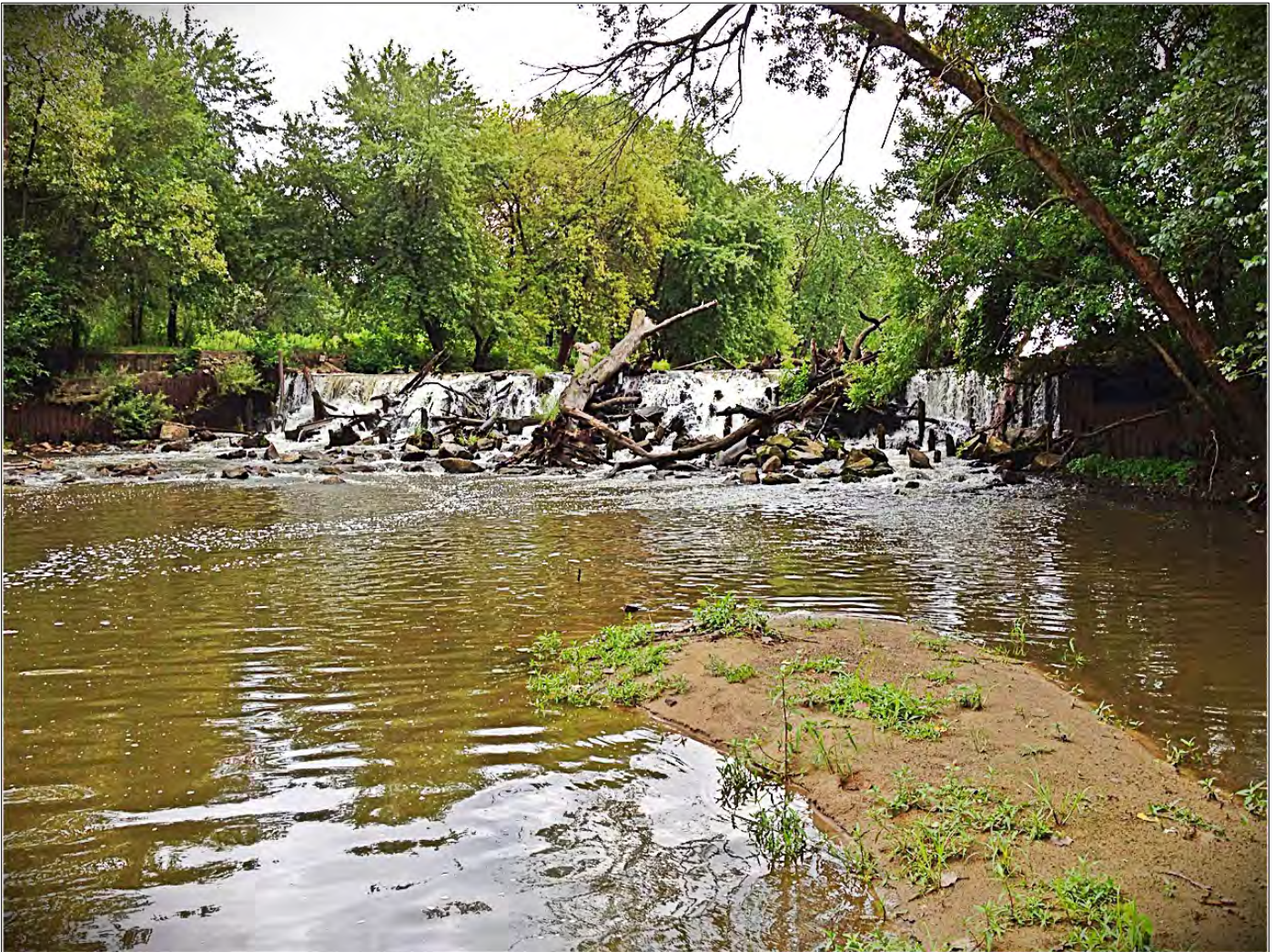
Figure 24 Deep River Dam
