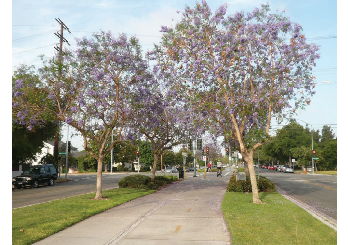
Shared use path in street median
