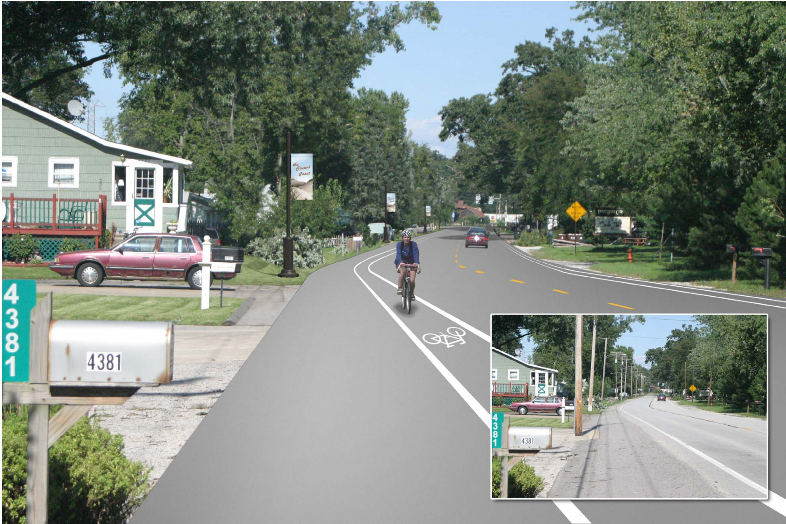
Figure 19 – US-12 Two-Lane with Bike Lane
