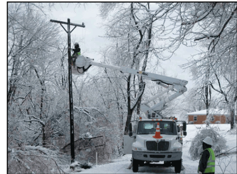
IBEW helps restore power after an Indiana ice storm, Source: ibew.org
