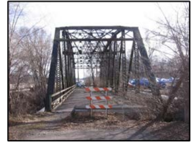
Old Crisman Road Bridge
