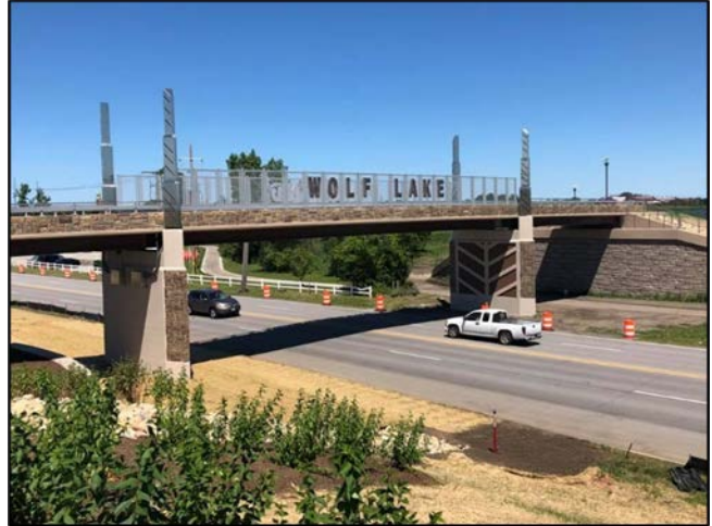
Wolf Lake Bridge in Hammond
