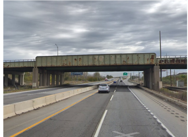
Former railroad bridge over Indiana Toll Road in Gary
