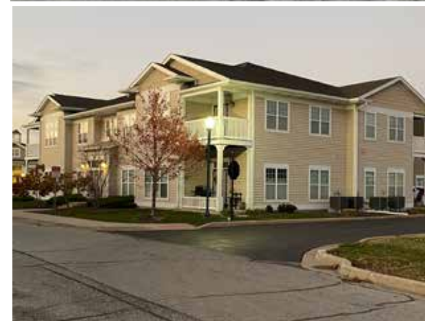
Innovative Urban Development Forms. From top: Townhomes in East Chicago, Street-oriented apartments in the Village at Burns Harbor.
