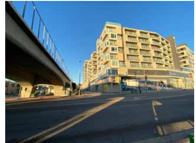
Transit oriented development outside of a city center. Along the Expo Line light rail in Los Angeles.
