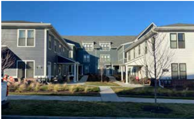
Bungalows at Prairie Queen (multifamily): Gross density – 23 du/A
