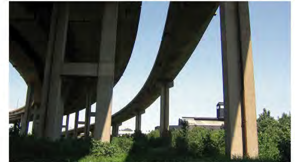
Elevated section of Cline Avenue over Indiana Harbor Ship Canal
