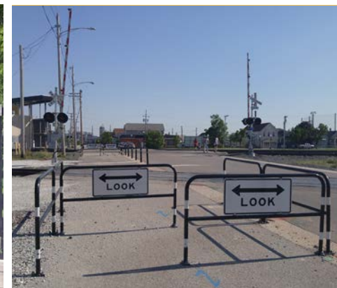
Protected crossings at railroad tracks in Whiting
