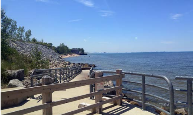
Beach closed due to sand erosion ▼
