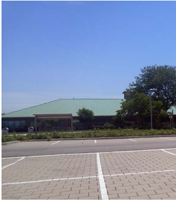
▲ Permeable pavement at Portage Lakefront and Riverwalk overflow parking lot
