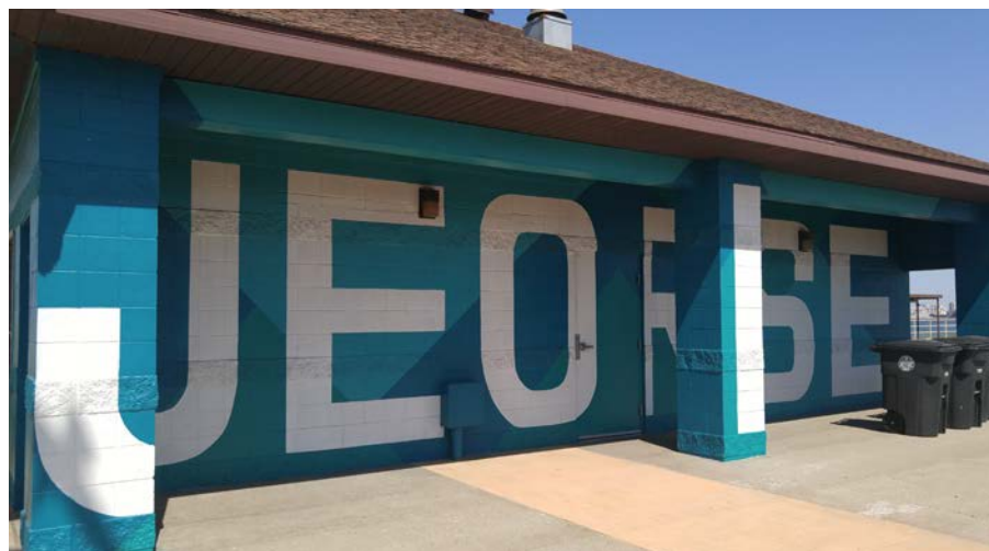
Public beach facilities and shelter at Jeorse Park and Beach
