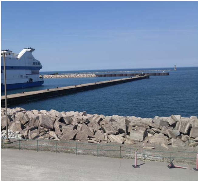
Majestic Casino breakwater ▲
