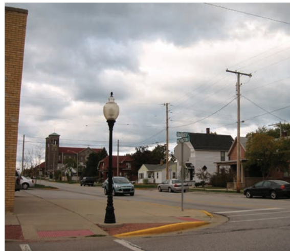
Sidewalk Infrastructure West Side, Michigan City (NIRPC)
