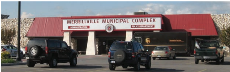
Merrillville Municipal Complex (NIRPC)
