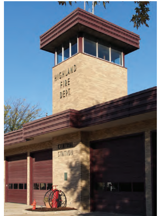
Highland Fire Station Downtown Highland (NIRPC)
