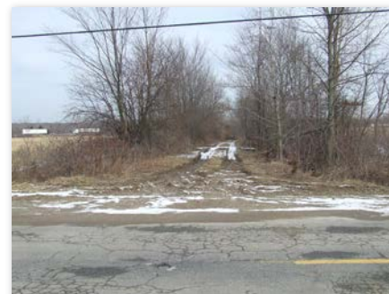
26 East looking north at Prairie alignment, just south of I-94
