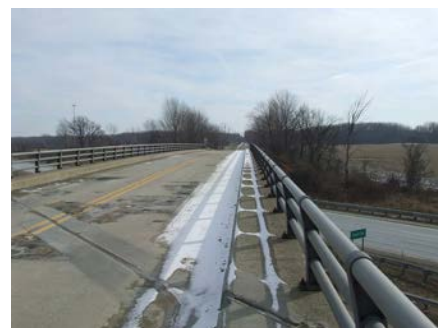
25 East at I-94 Bridge
