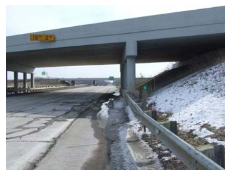
34 US-12 @ I-94 looking east
