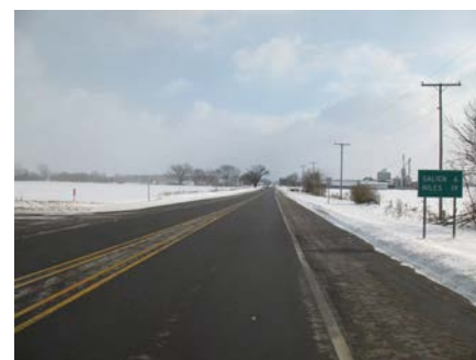
41 US-12 East of Three Oaks looking east
