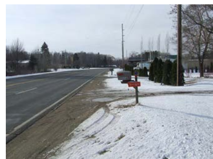
19 Red Arrow Near Parkway
