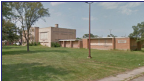
POTENTIAL ADAPTIVE REUSE SITES: 475 BROADWAY (TOP), HISTORIC BROADWAY BUILDINGS (CENTER), AMBRIDGE SCHOOL (BOTTOM)
