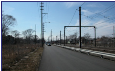
SOUTH SHORE RAIL LINE LOOKING WEST
