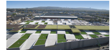
GREEN ROOFS AND PERMEABLE PAVERS CAN SIGNIFICANTLY RETAIN SURFACE RUNOFF AND REDUCE THE NEED FOR ONSITE WATER STORAGE.
