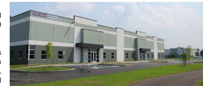
6340 AMERIPLEX DRIVE IN AMERIPLEX AT THE PORT
