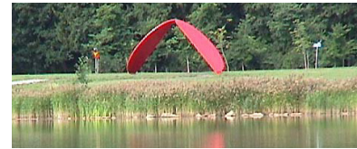
I- 80/94 BRIDGE ENHANCEMENT AND PUBLIC ARTS CAN ADD TO VIBRANCY OF THE CORRIDOR
