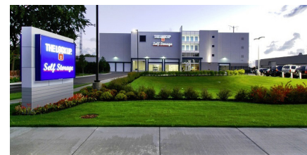
FRONTAGE LANDSCAPING AND SETBACK CAN REDUCE THE IMPACT OF THE USE ON SURROUNDING AREAS.
