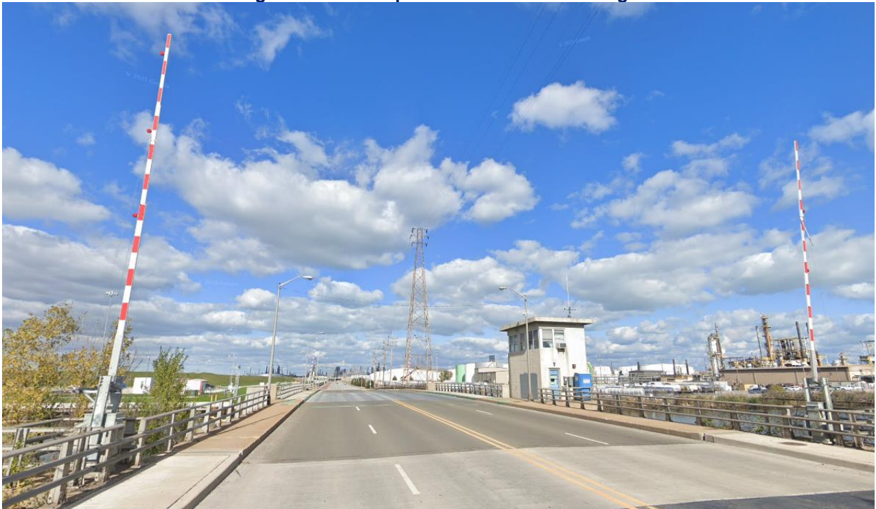
Figure 43: Indianapolis Boulevard Drawbridge
